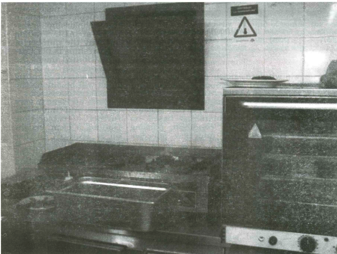
A cooker hood is needed to capture the smells and grease in the kitchen and around the outlet
